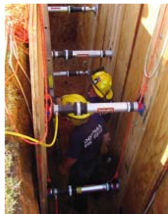
Trench shoring with pneumatic Auto-lock struts.
