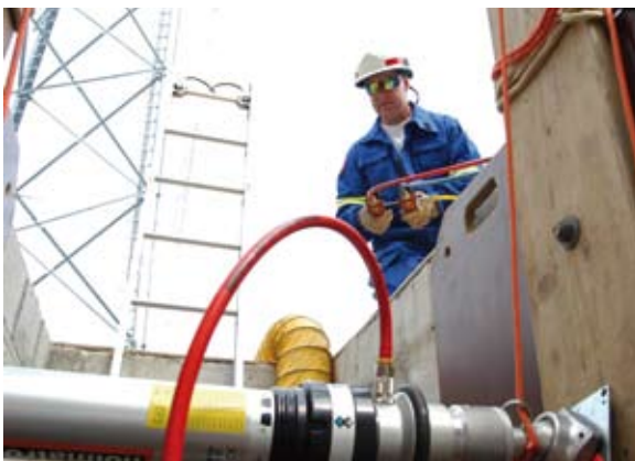
Remote shoring of a trench.
